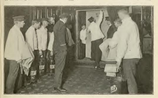
CLOSING A FIRE BULKHEAD ABOVE THE WATERLINE Stewards are Drilled to use Fire Pails and Wet Blankets
