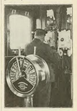
The Engine Telegraphs are on the Bridge and other Parts of the Vessel
